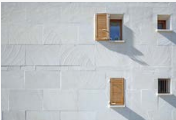
© Perraudinarchitecture (S. Demailly), Cornebarrieu (31), ZAC Monges
