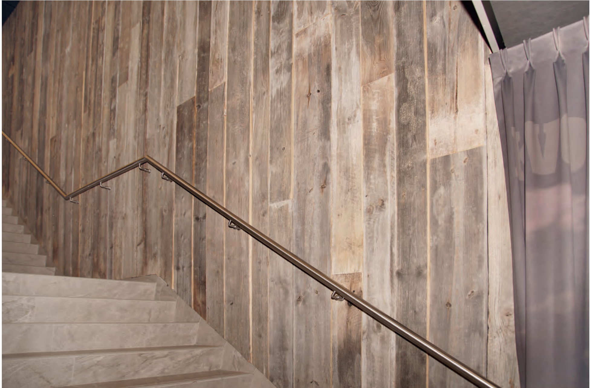
project: KVO, Oostende | hout: Reclaimed, Europees Barnwood | uitvoerder: Laco Projectflooring & Finishing | architect: Steven Vernackt
